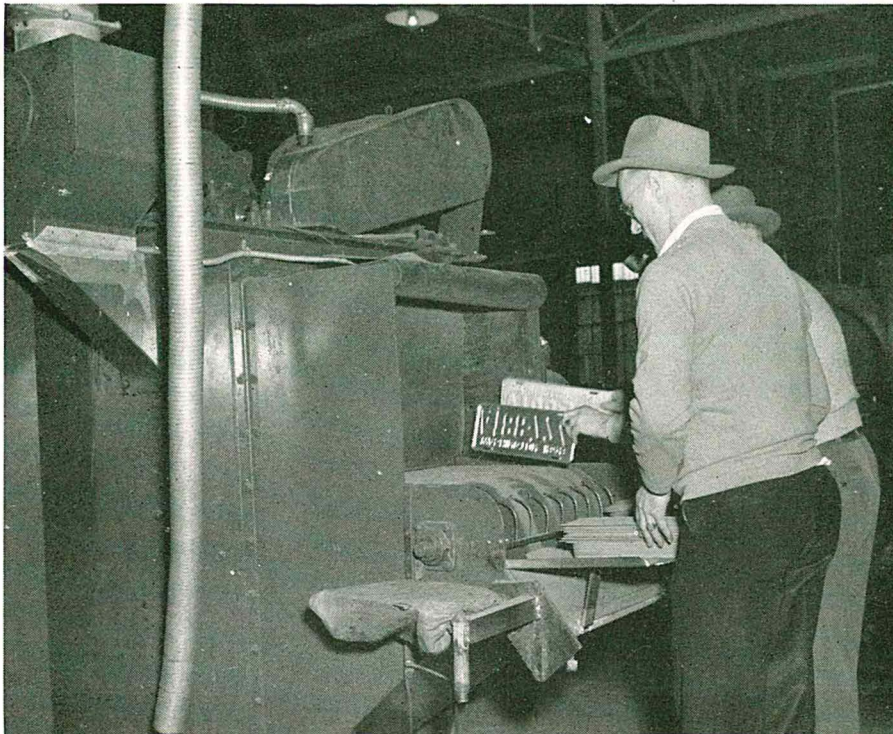
Unloading Wheelabrated license plates at Washington State Prison. Notice the dull, non-reflecting surface of the front side of the license plate the farthest from the camera. This dull surface enables the plate to be seen at night without glare, and provides a bond for the paint.
